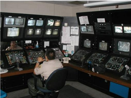
Also located in the Main Jail, is the main control room. Here one or two staff controls all access doors and elevators. All security systems and fire alarms are also controlled here. This is an extremely busy area during most of the day and night and only slows down briefly during early morning hours.
