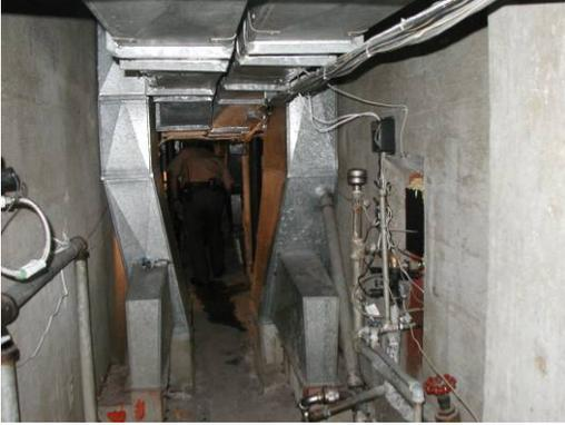
During the on-site visit, a freshwater plumbing line burst in this cell chase. This line was encased in concrete and required many staff hours to repair – during which time all water to the cells in this block were cut off. With water unavailable the inmates were unable to flush their toilets. Should there have been complications to this situation, the inmates would have needed to be moved to another space – a very difficult and time-consuming process given
