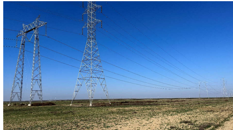
Photograph 8. View of the Parcel 085-040-36S and the electrical transmission lines along the eastern boundary.
