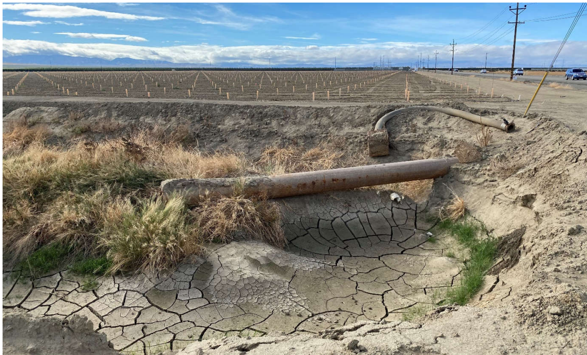
Photograph 8. Dry tailwater basin on northeastern portion of Project site adjacent to active agriculture area. View west. November 9, 2021.
