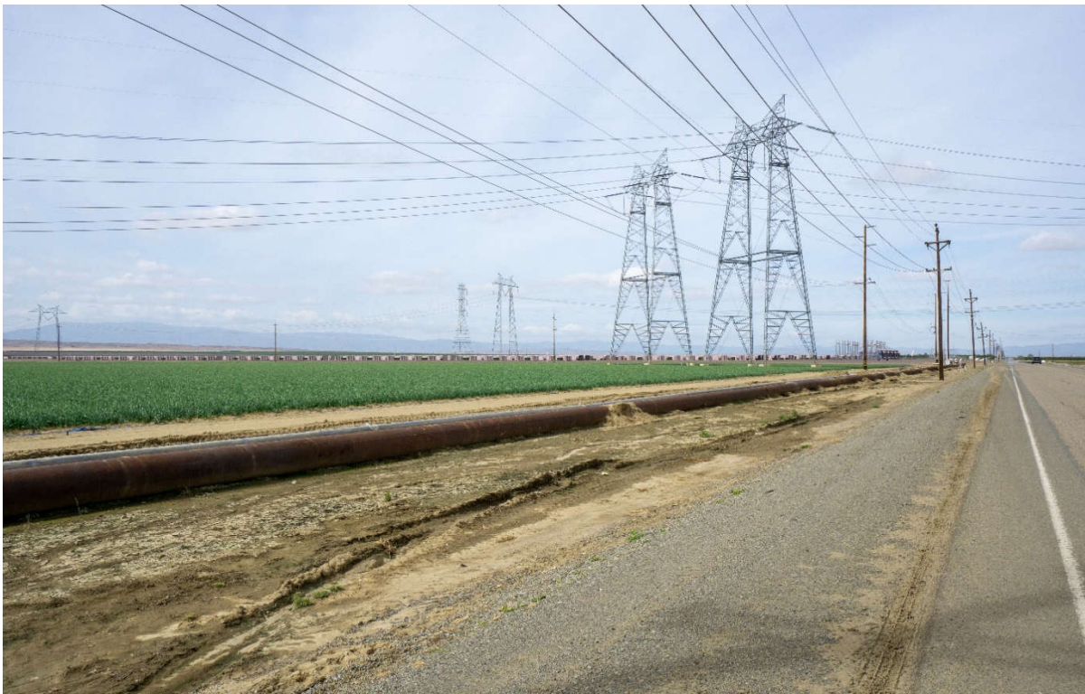
Photograph 2. Simulated view after construction of the proposed lithium-ion battery option.
