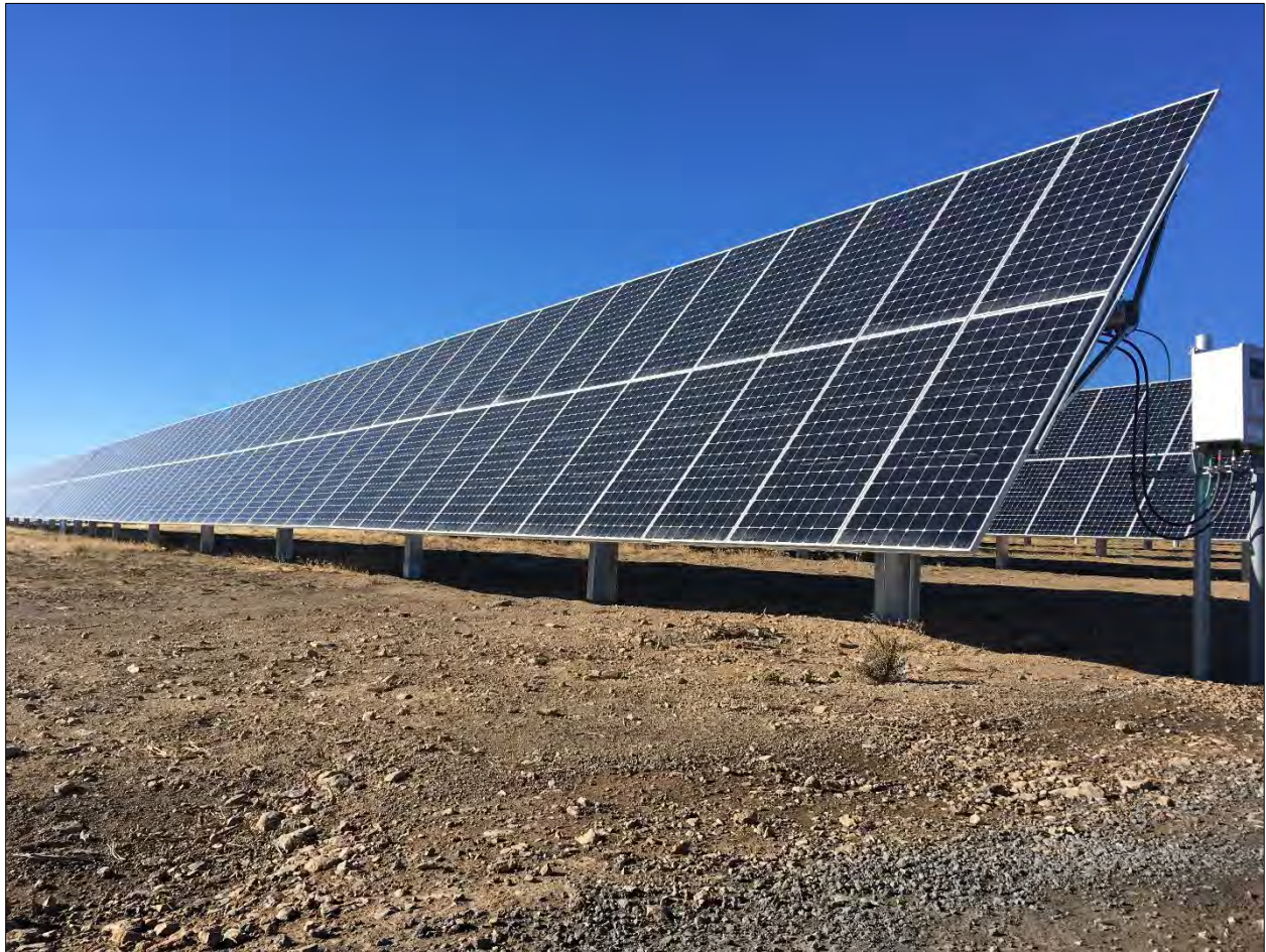
Figure 3. Typical Tracker Panel and Pier Design
