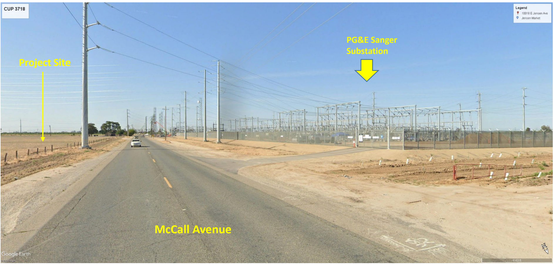
Project Site Steet View – Looking South
