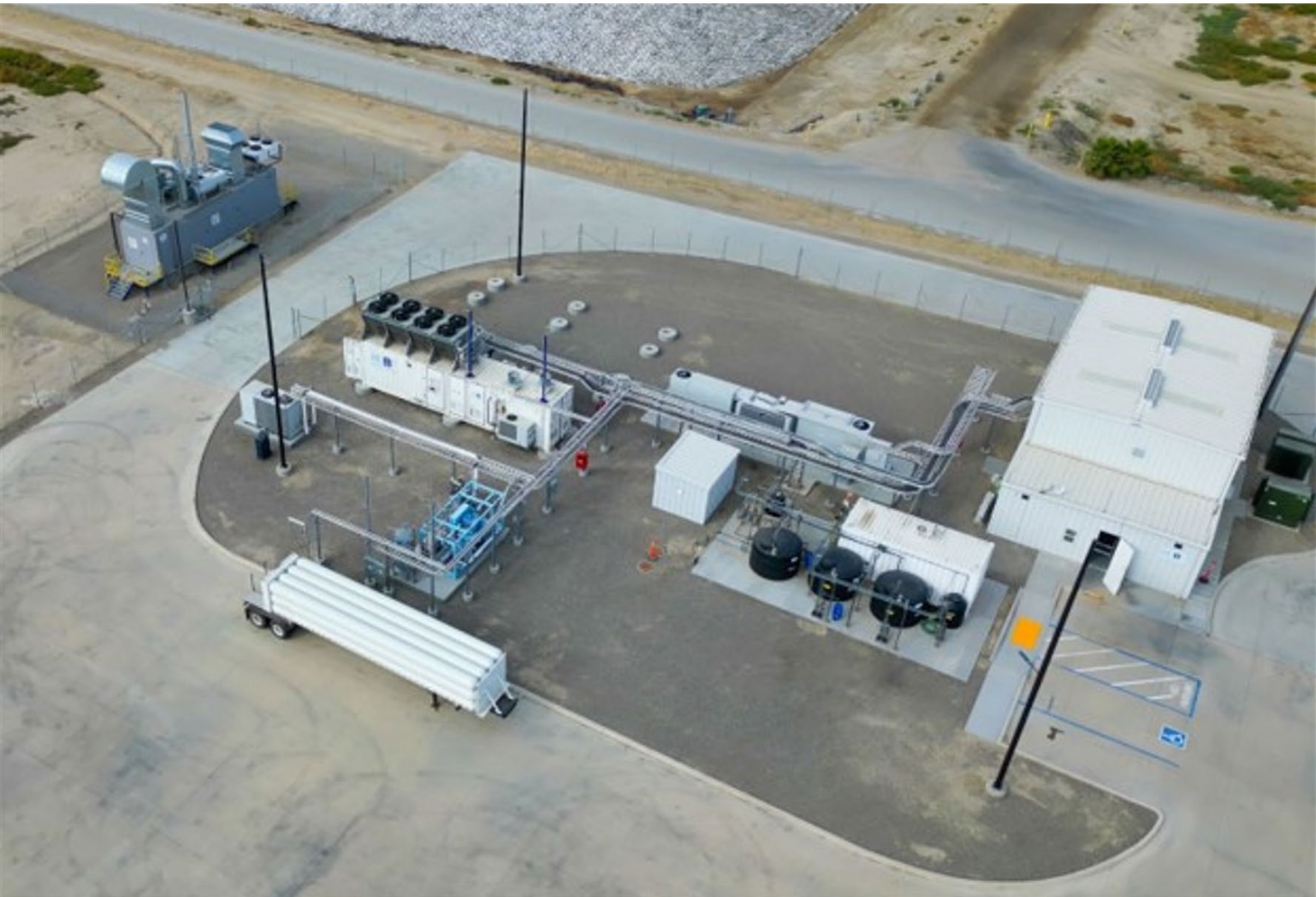
Hydrogen facility site aerial – looking southwest
