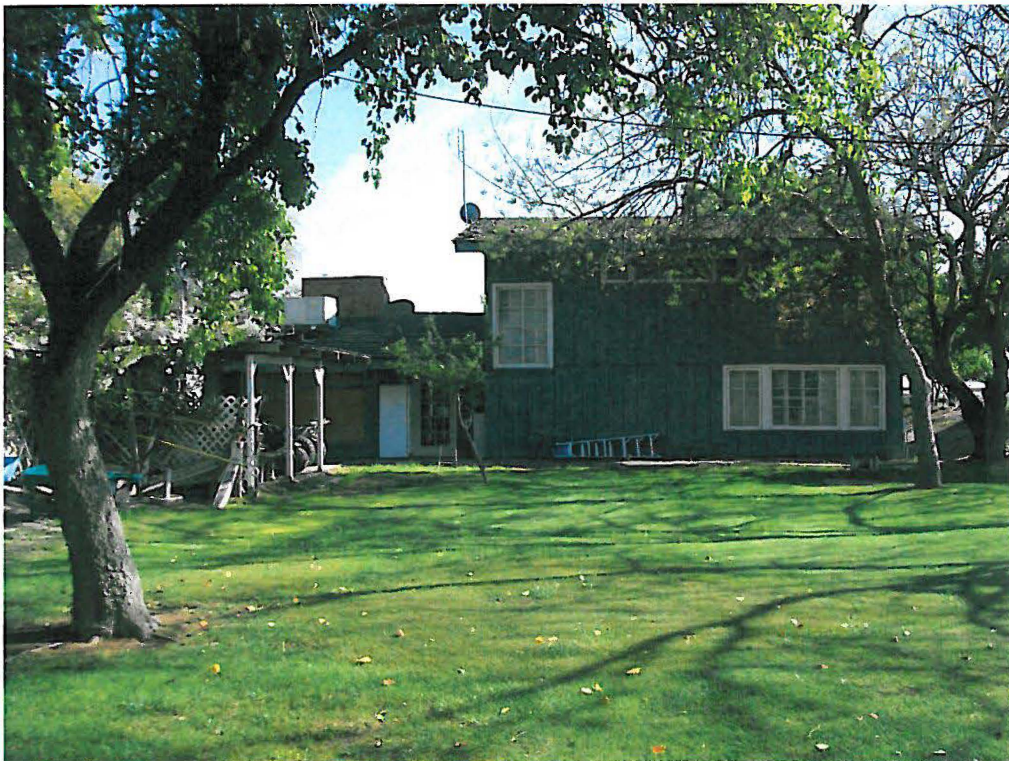
Photo 4: Southern-facing view of the on-site dwelling.
