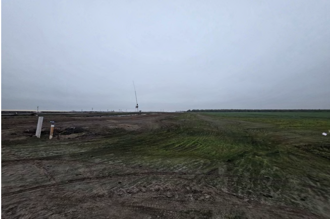
Figure 9: Southeast corner of future wastewater processing beds area.
