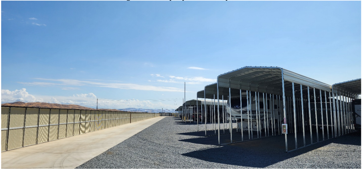
Looking East from proposed facility location
