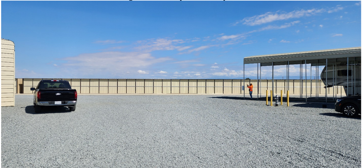
Looking North at Proposed facility location
