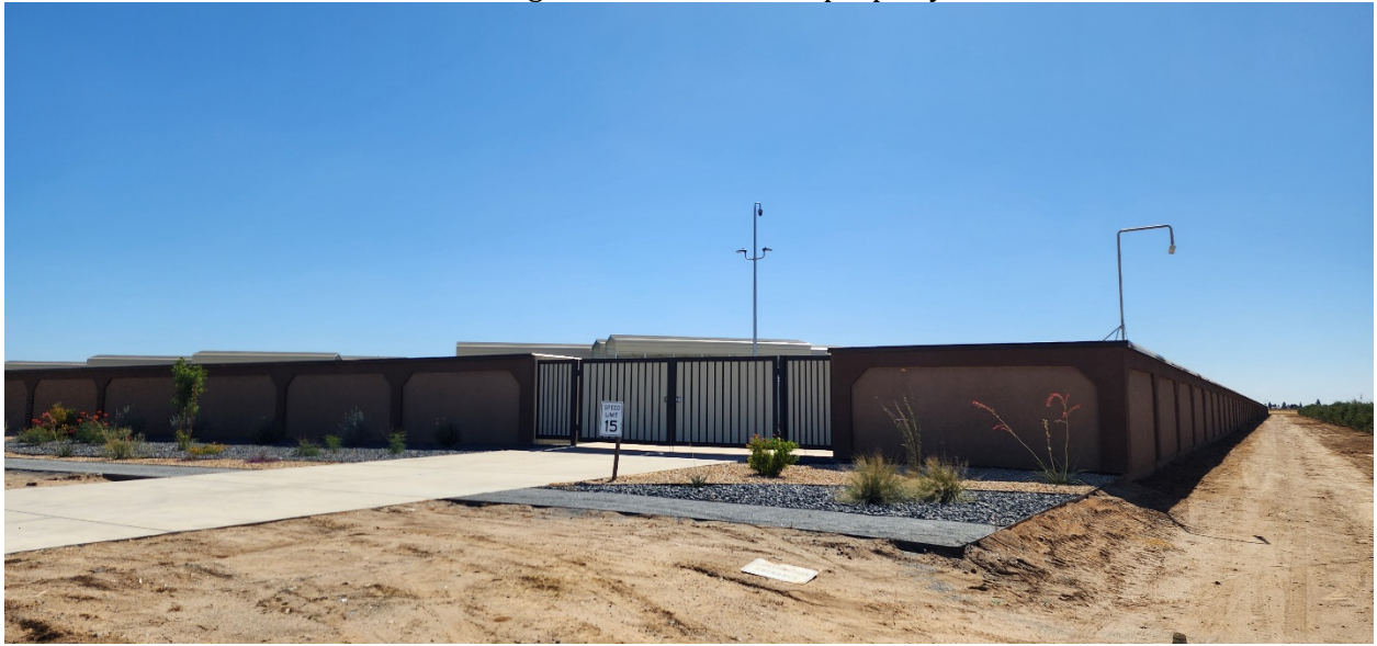
Looking Southwest towards property
