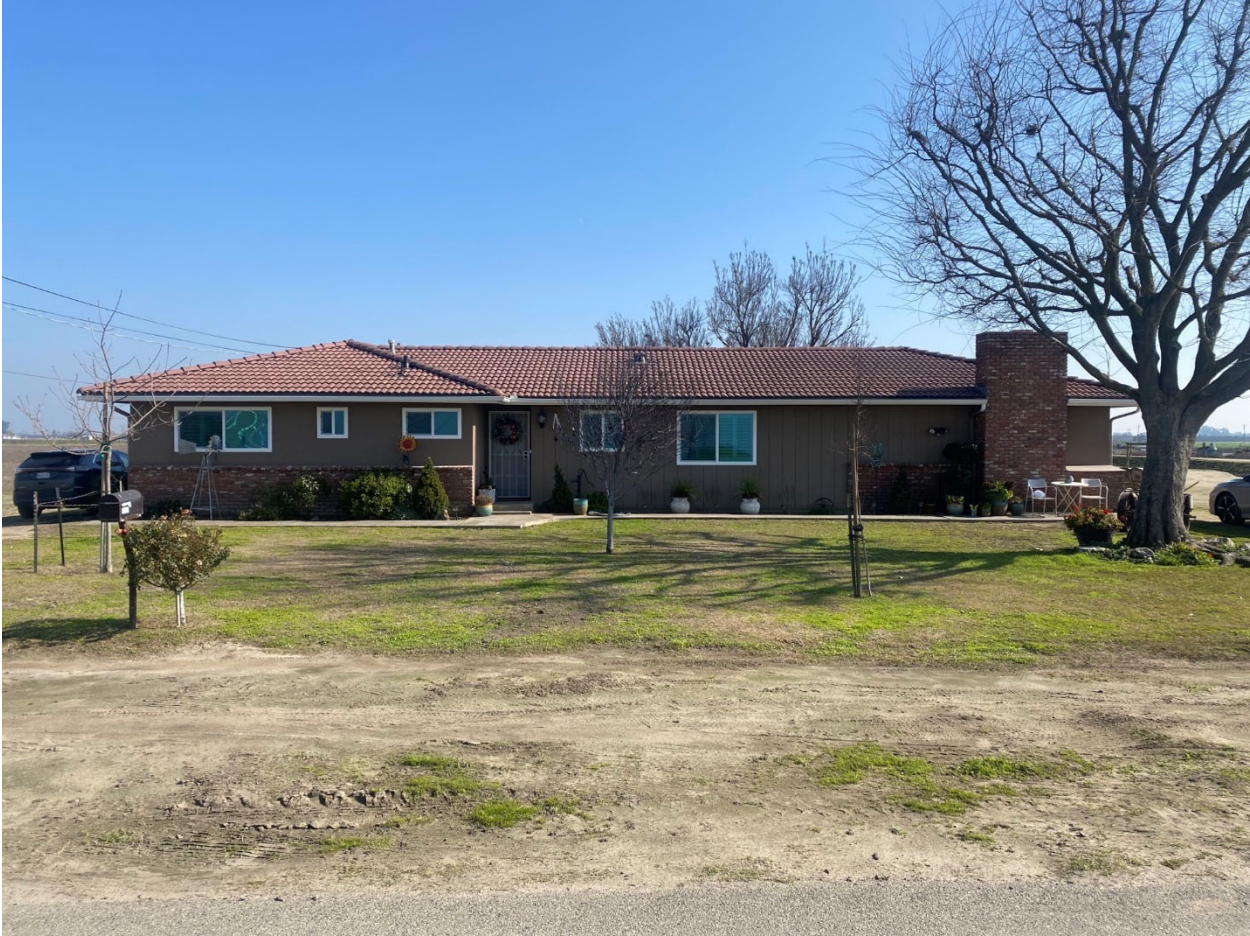
WEST SIDE OF RESIDENCE
