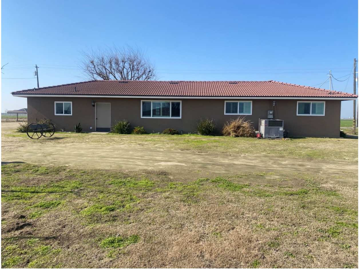
EAST SIDE OF RESIDENCE
