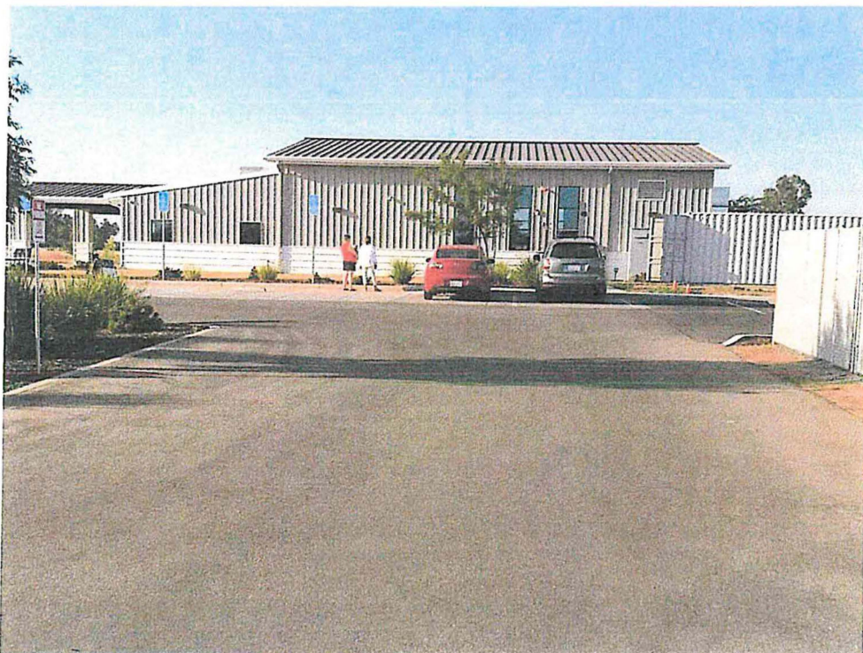
NORTH SIDE VIEW OF EXISTING BUILDING
