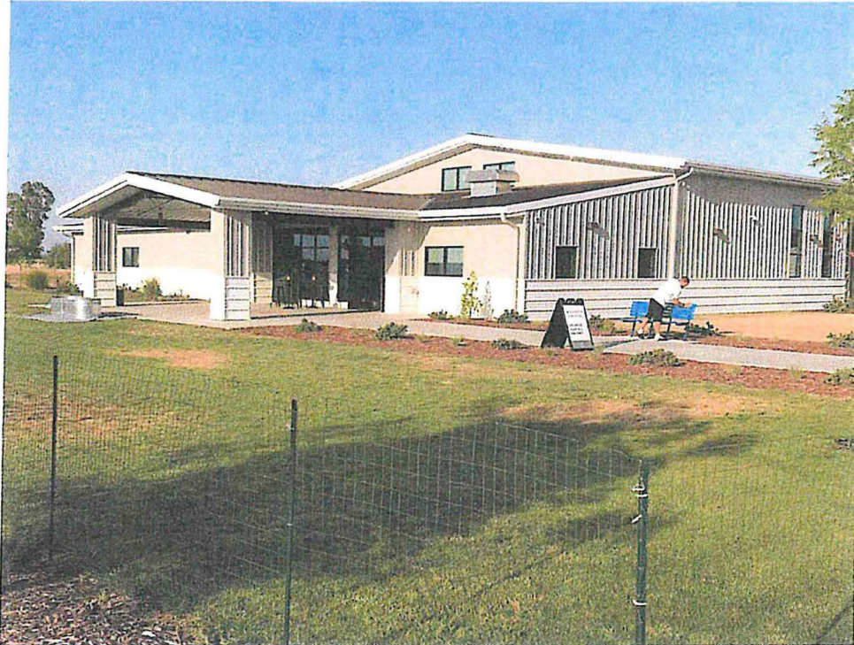
NORTH EAST SIDE VIEW OF EXISTING BUILDING
