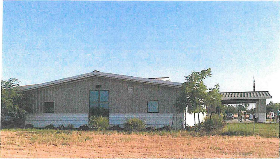
SOUTH SIDE VIEW OF EXISTING BUILDING
