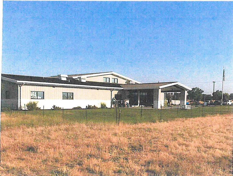
EAST SIDE VIEW OF EXISTING BUILDING
