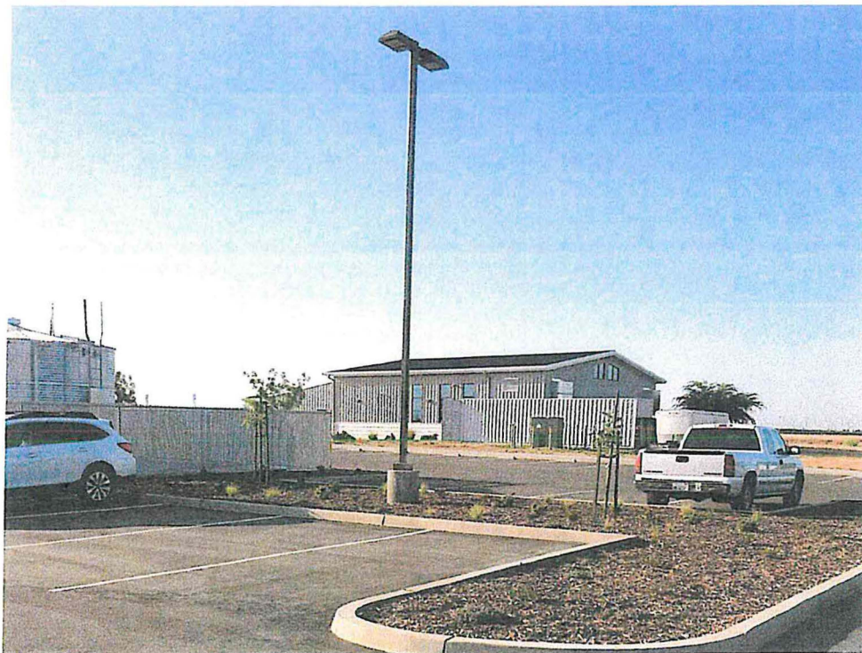
NORTH WEST SIDE VIEW OF EXISTING BUILDING
