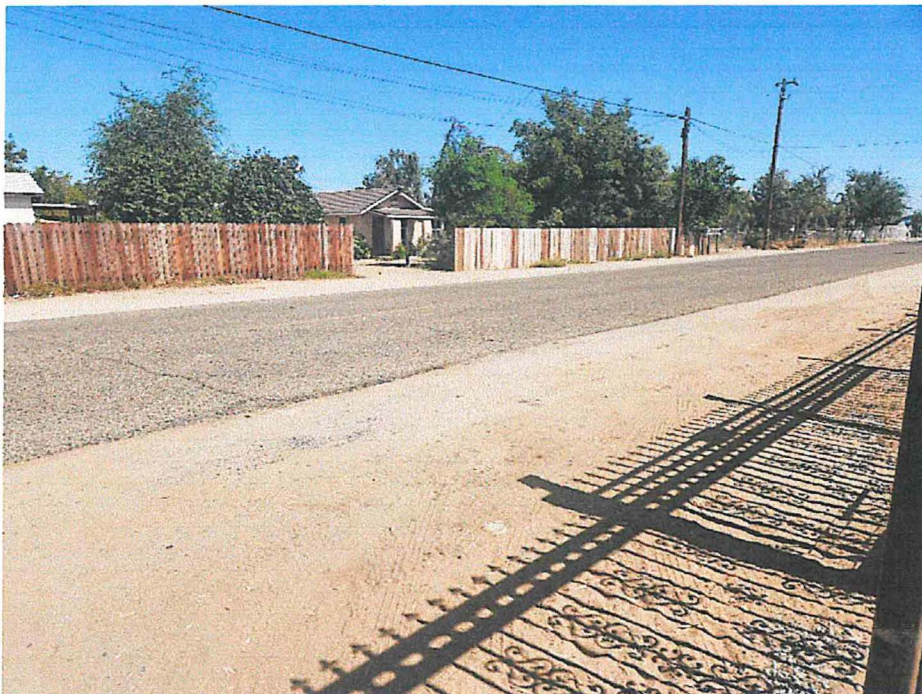
Looking northeast from front of property @ W. Church Ave.
