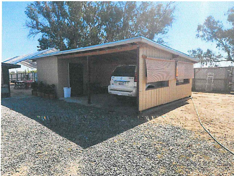
Existing detached structure from the northwest
