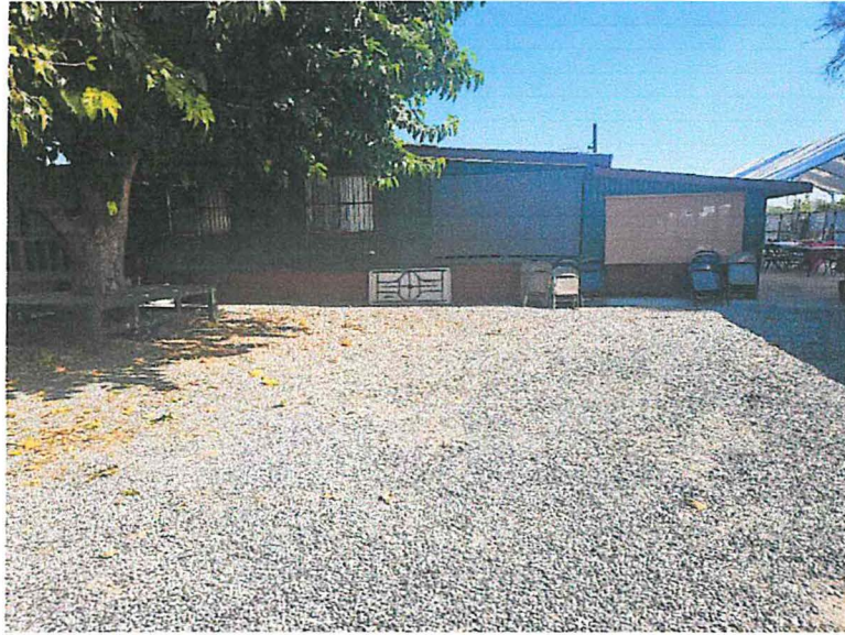
Existing residence from the north
