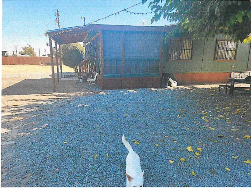
existing residence from the west
