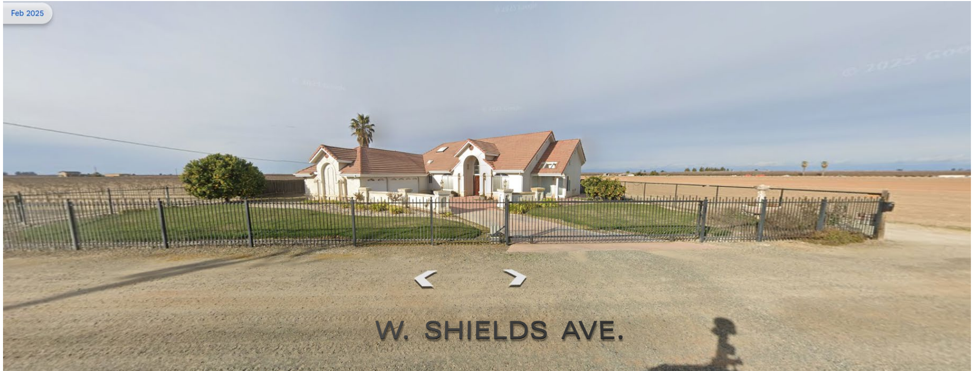
STREET VIEW LOOKING NORTHWARD FROM SHIELDS AVE
