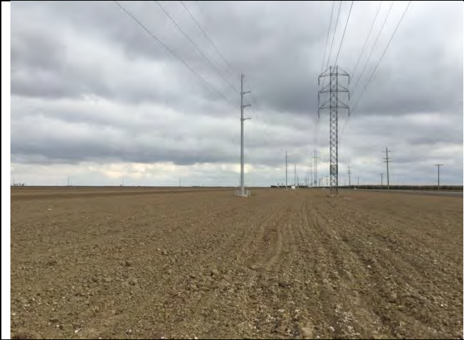
Photo 13. Looking east from the west along transmission line.
