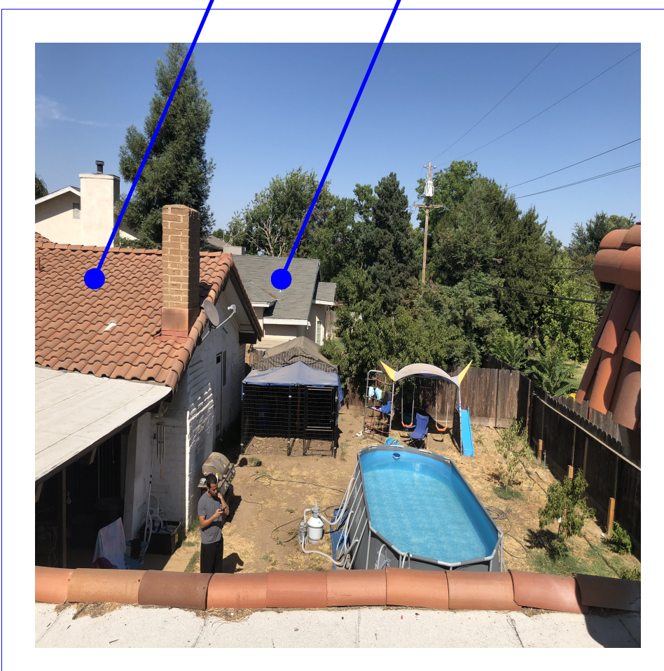
VIEW FROM ROOF OF ACCESSORY TOWARD EAST : applicant's rear landscape and neighbor rear yard beyond
