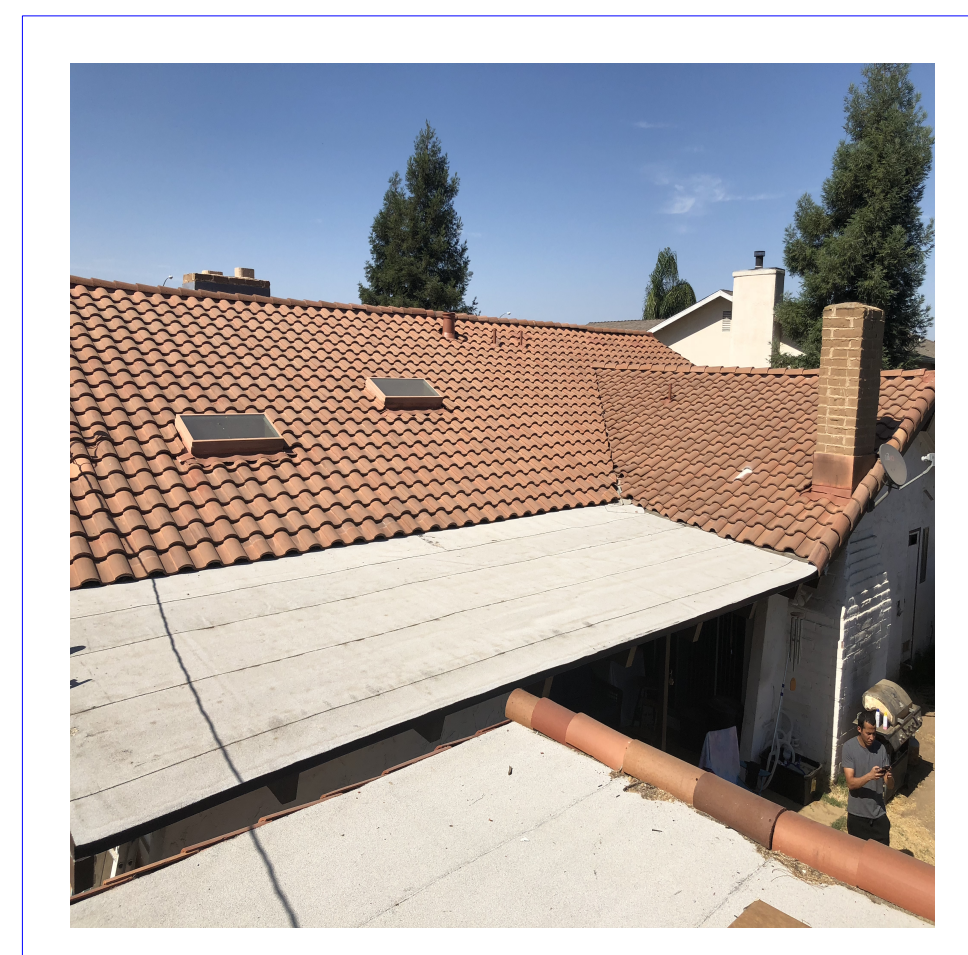
VIEW FROM ROOF OF ACCESSORY TOWARD NORTHEAST : applicant's house
