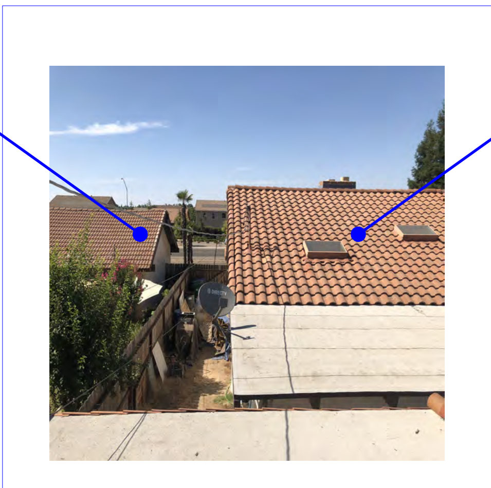
VIEW FROM ROOF OF ACCESSORY TOWARD NORTH applicant and adjacent roofs
