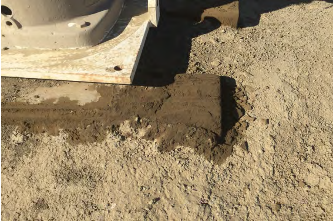
Site 4: Soil staining around base of ag pump.
