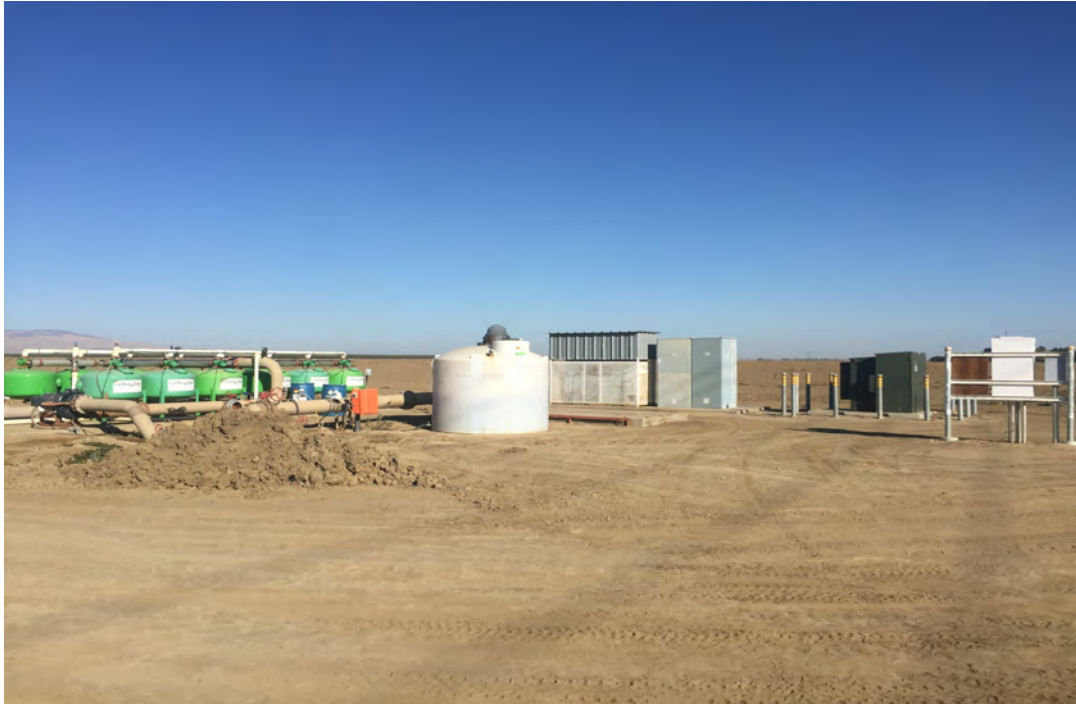
Site 1: Adjacent property. See site notes.
