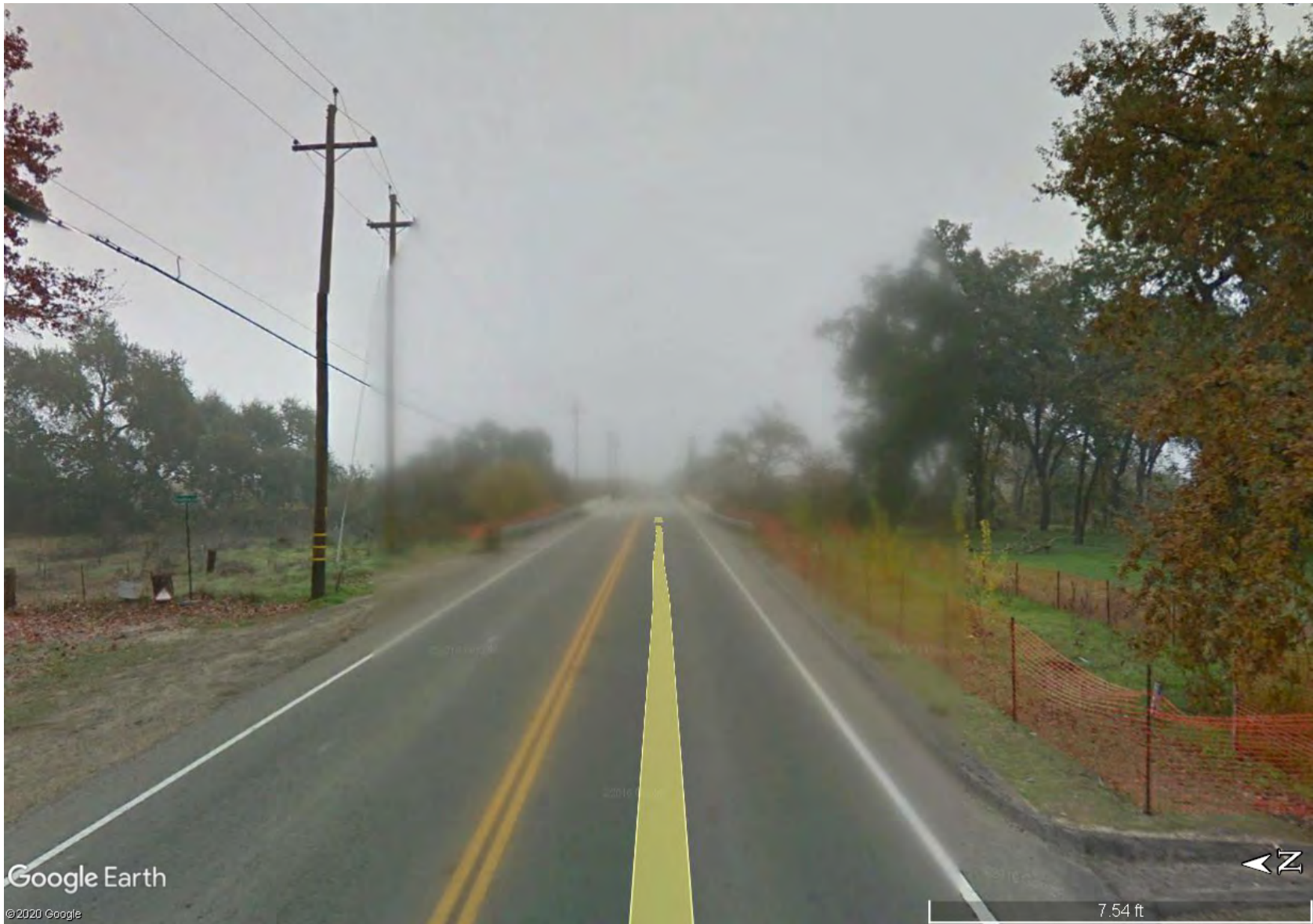
Figure 12 – E Goodfellow Avenue facing east towards the bridge structure over the Bryd Slough.
