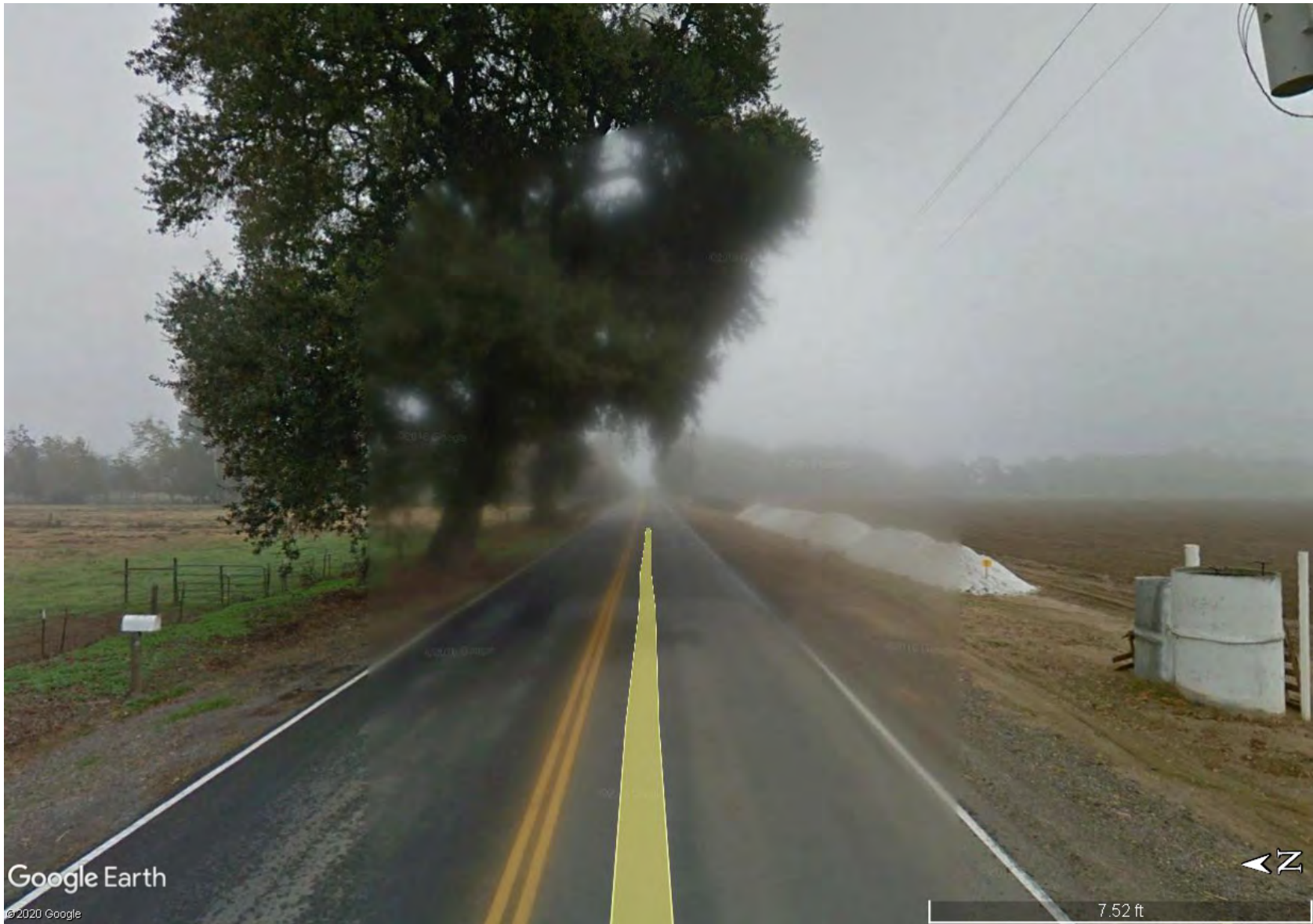
Figure 11 – E Goodfellow Avenue from approximately 100 feet east of the E Goodfellow Avenue and S MacDonough Avenue intersection.
