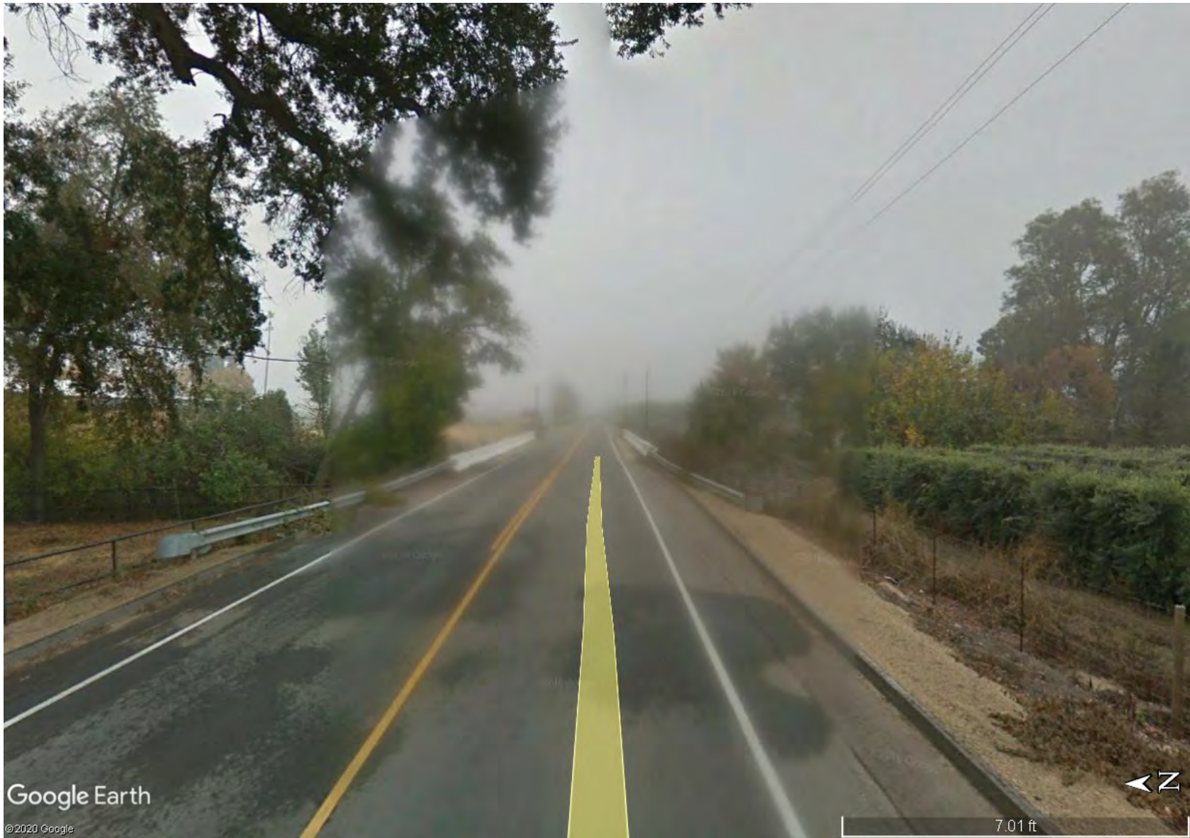
Figure 8 – E Goodfellow Avenue facing east towards the bridge structure over Cameron Slough.
