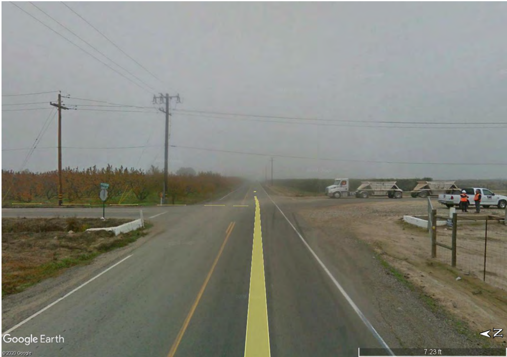
Figure 6 – E Goodfellow Avenue facing east towards the E Goodfellow Avenue and S Riverbend Avenue intersection and Hanke Ditch.
