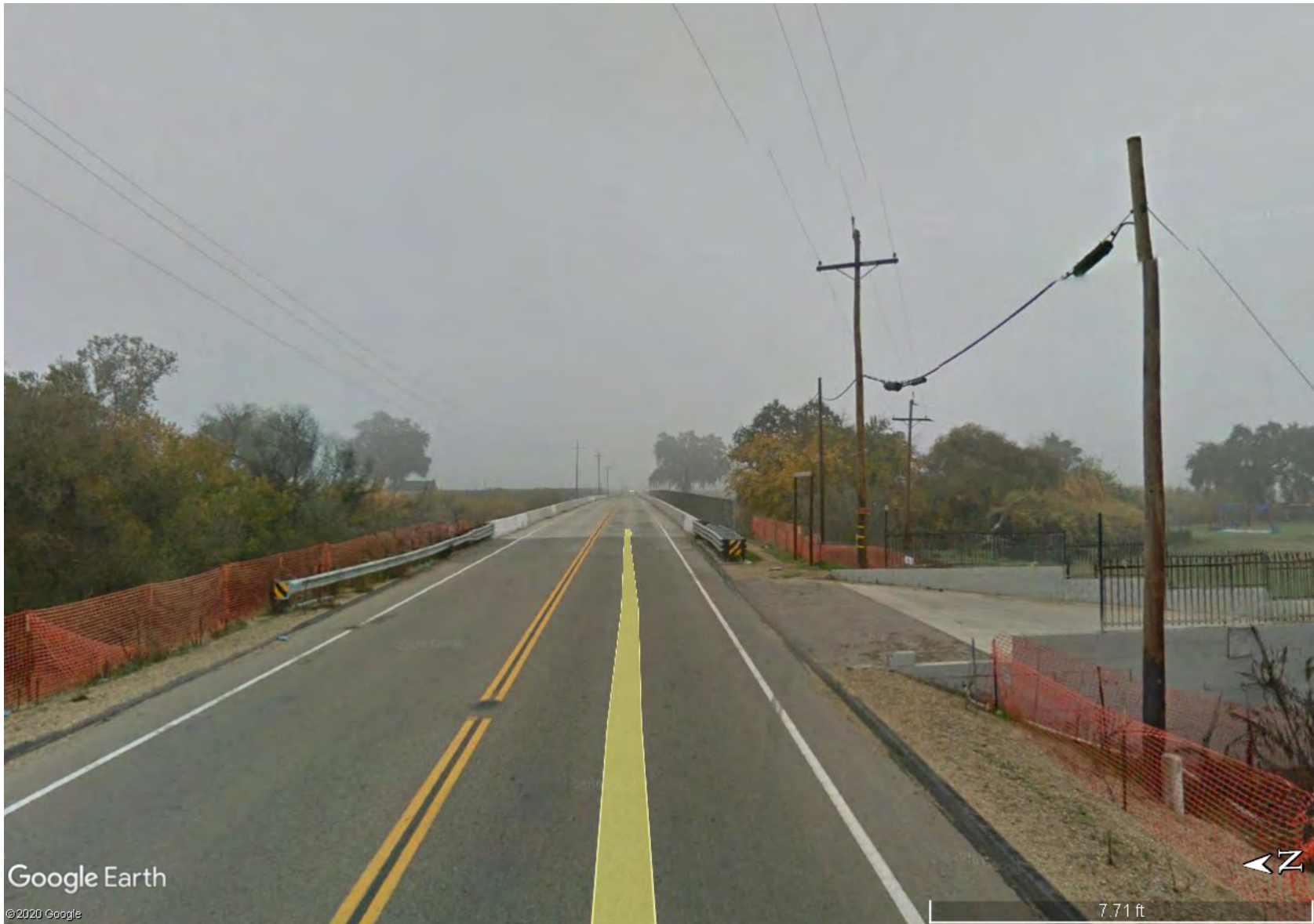
Figure 2 – E Goodfellow Avenue facing bridge structure over the Kings River.
