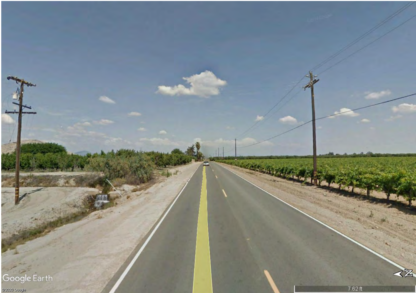
Figure 20 – E Goodfellow Avenue from approximately 520 feet of the E Goodfellow Avenue and Jim Savage Road T-Intersection.
