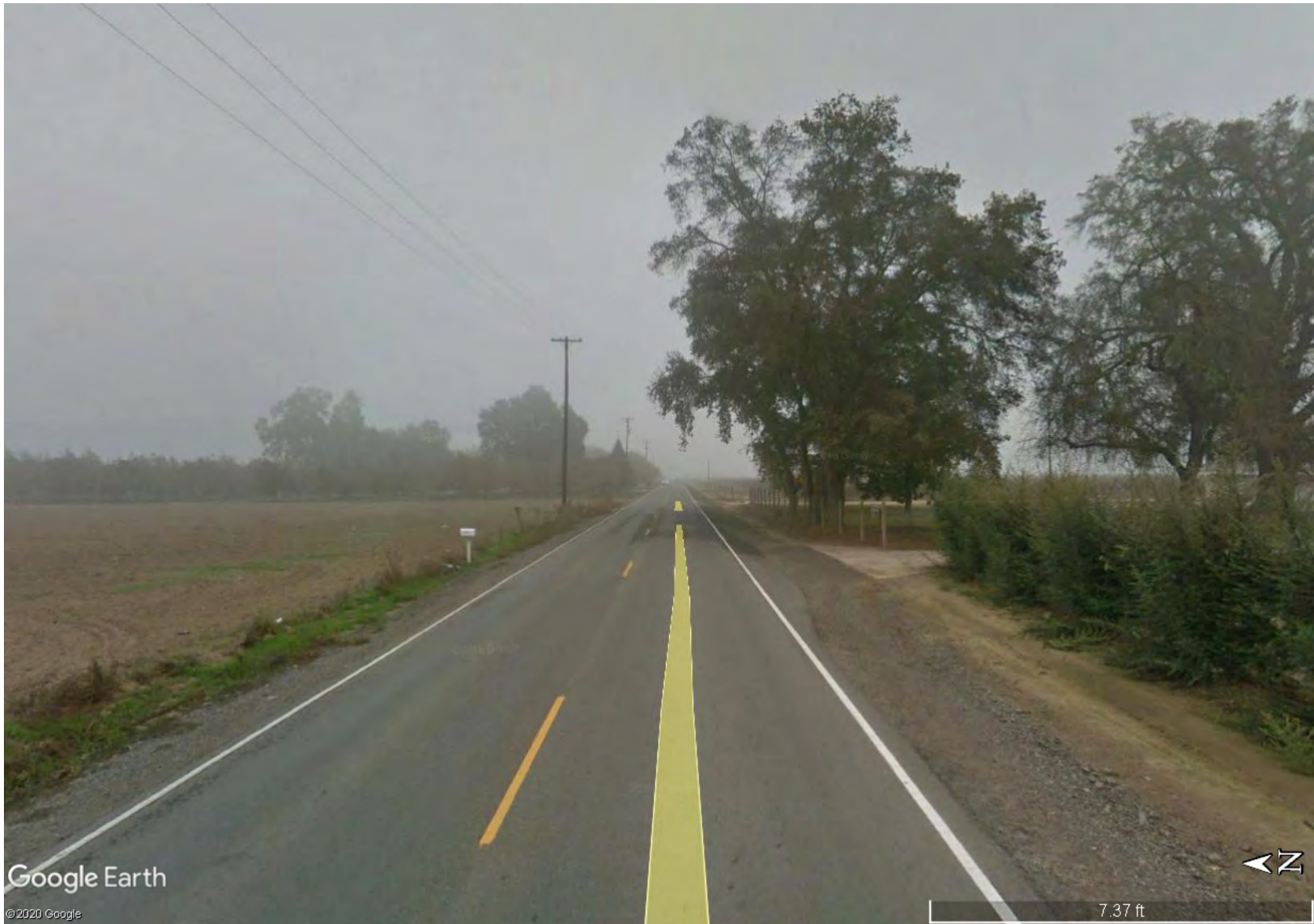
Figure 5 - E Goodfellow Avenue facing east from 15211 East Goodfellow Avenue, Sanger, CA 93657.
