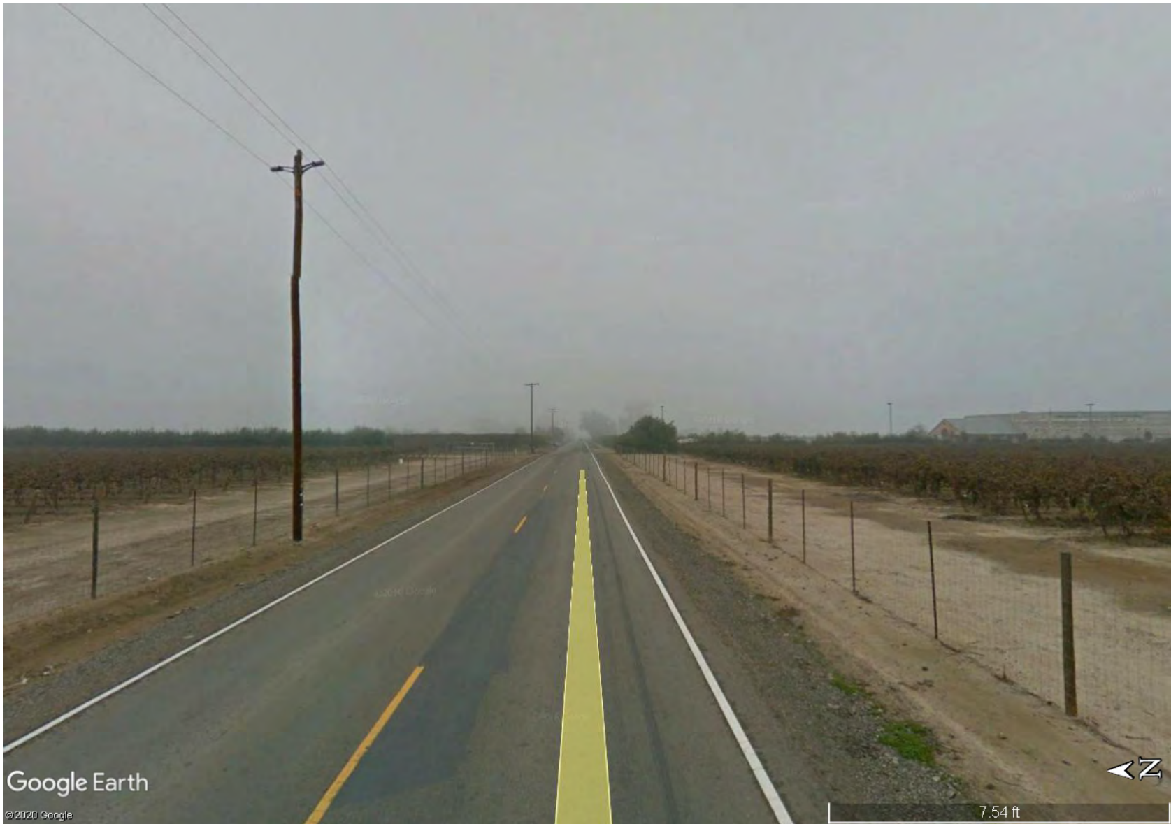
Figure 4 – E Goodfellow Avenue facing east from 14865 East Goodfellow Avenue, Sanger, CA 93657.
