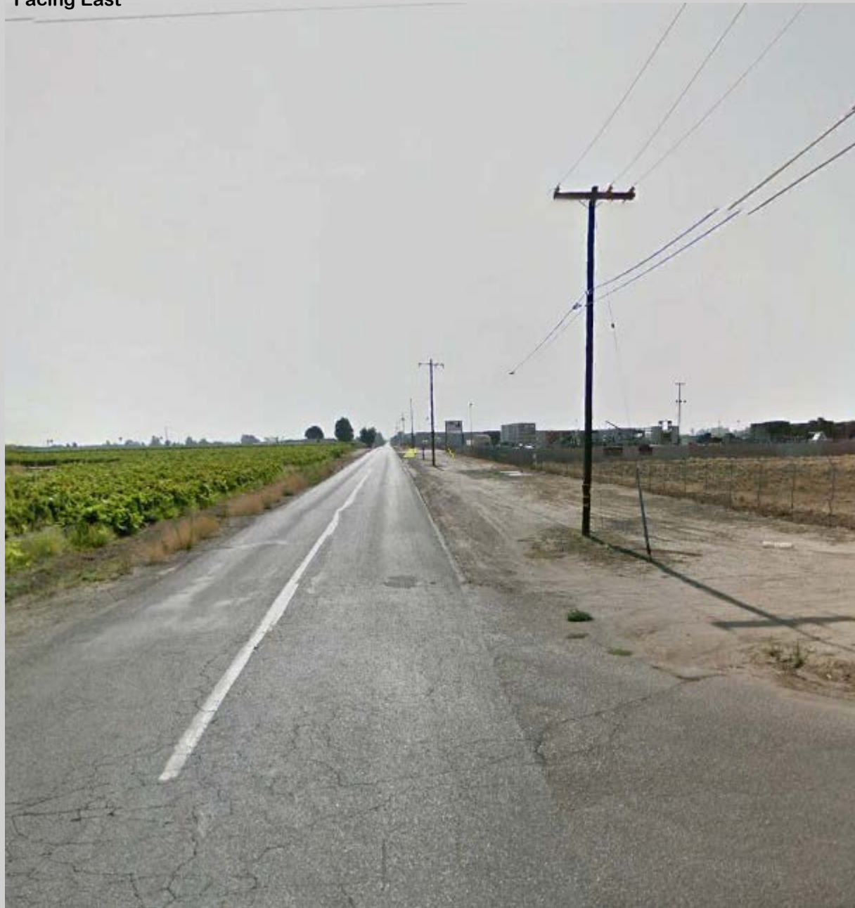
American Avenue Facing East
