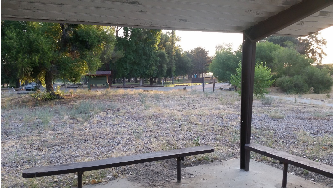
Photo 1 Existing Picnic area - ADA Trail Area
