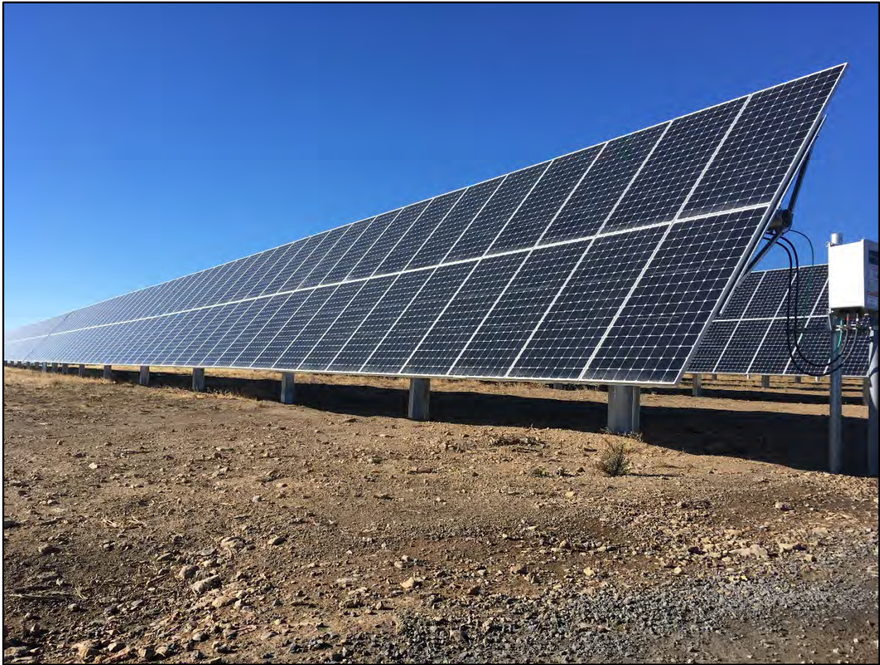
Figure 4. Typical Tracker Panel and Pier Design
