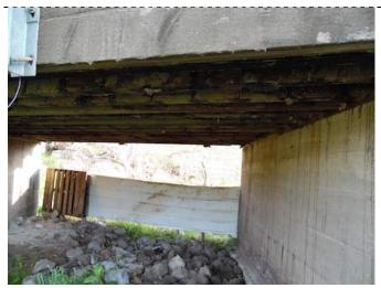
$\underline{Photograph\ B5}$  – Timber undercarriage of bridge, and fencing blocking channel for livestock preservation.
