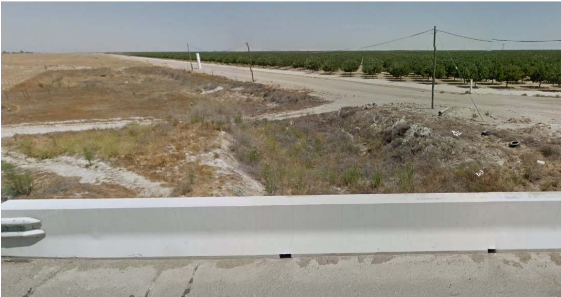
Figure 7: East branch looking downstream at existing access road crossing channel
