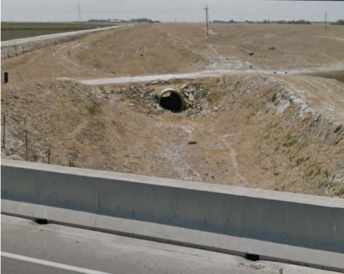
Figure 6: East branch looking upstream at existing access road and culvert
