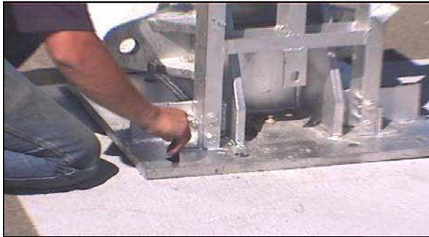
Use the Base Plate of the Compact Backstop as a template
