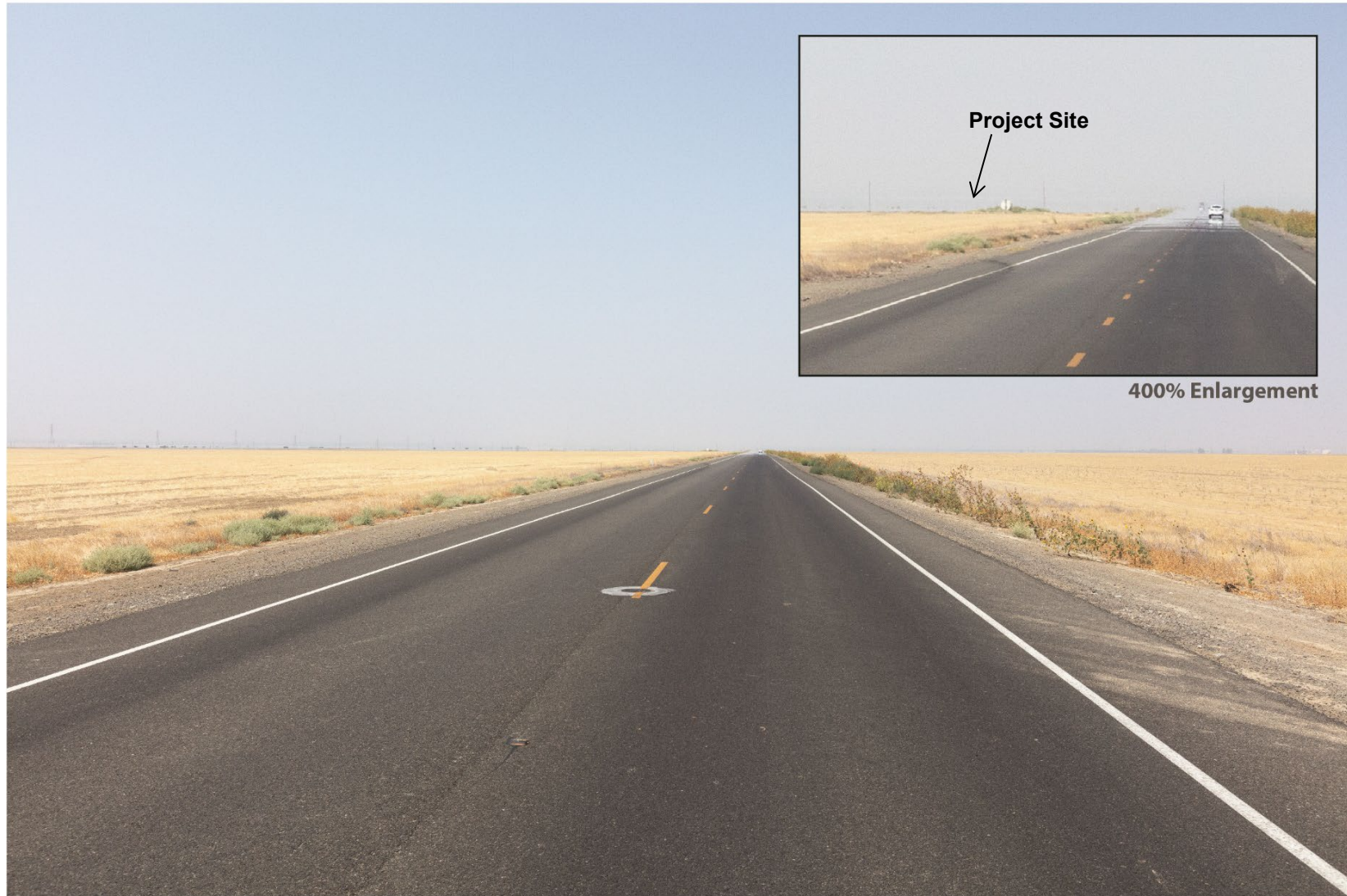
Figure 4.1-3 Existing View from KVP 2 Looking West along West Manning Avenue toward the Project Site
