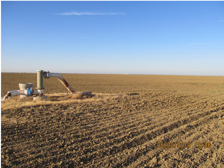
Photo 5. Looking northeast from Monterey Avenue 0.5 mile south of Manning Avenue
