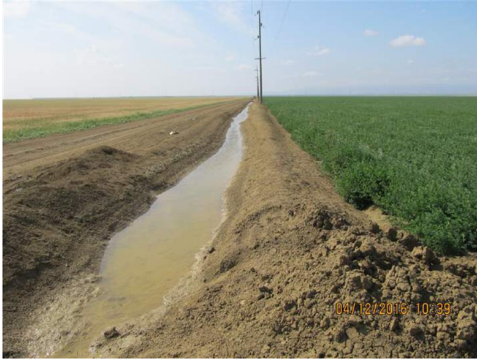
Photo 1. A temporary drainage ditch and alfalfa field typical of the south-center of the site.
