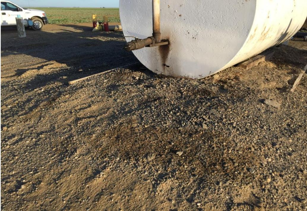
Site 1 (Figure 2): Soil staining near south side base of fuel AST located at southwest corner of APN 028-071-47T.
