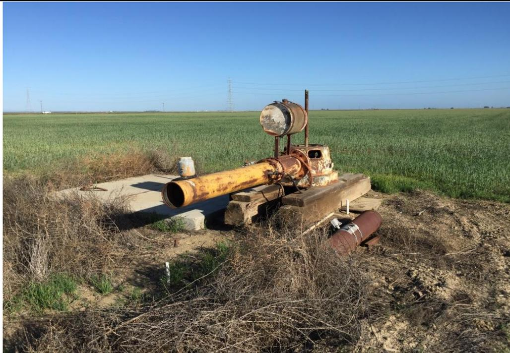
Site 4 (Figure 2): Agriculture pump, agriculture well and turbine oil tank. Well not in use. Staining around pump.
