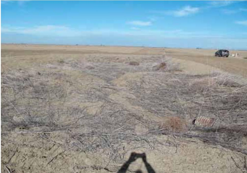
Close-up of storm water/tail water pond in northeast corner of Site. Corrugated metal pipe discharges water into pond, no outlet pipe in pond.
