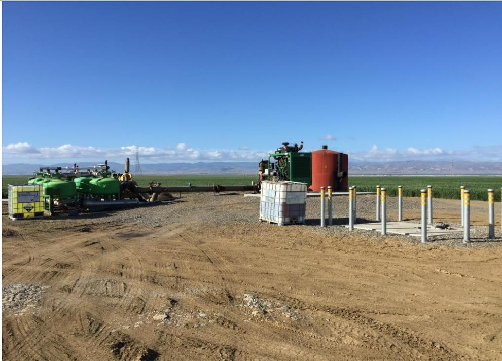
Site 6 (Figure 2): Adjacent property located south of APN 028-111-10T. Site contains agriculture well, agriculture chemical filtration station, agriculture pump with turbine oil tank, agriculture diesel engine with engine oil tank and AST.
