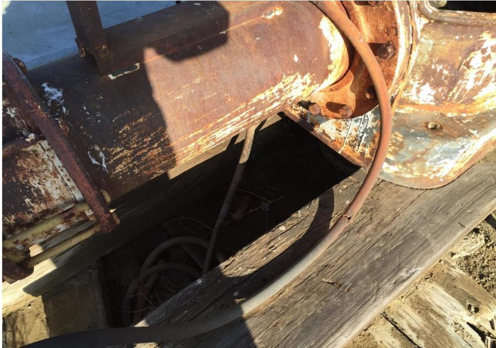
Site 4 (Figure 2): Agriculture pump, agriculture well and turbine oil tank. Well not in use. Staining around pump. Located east of the southwest corner of APN 028-111-01ST.
