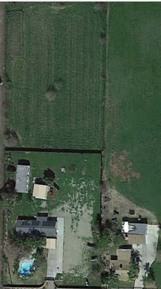
PG&E Reedley Substation
