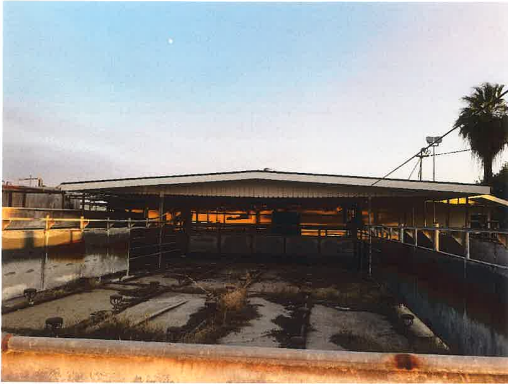
Image taken facing South of North side of building
