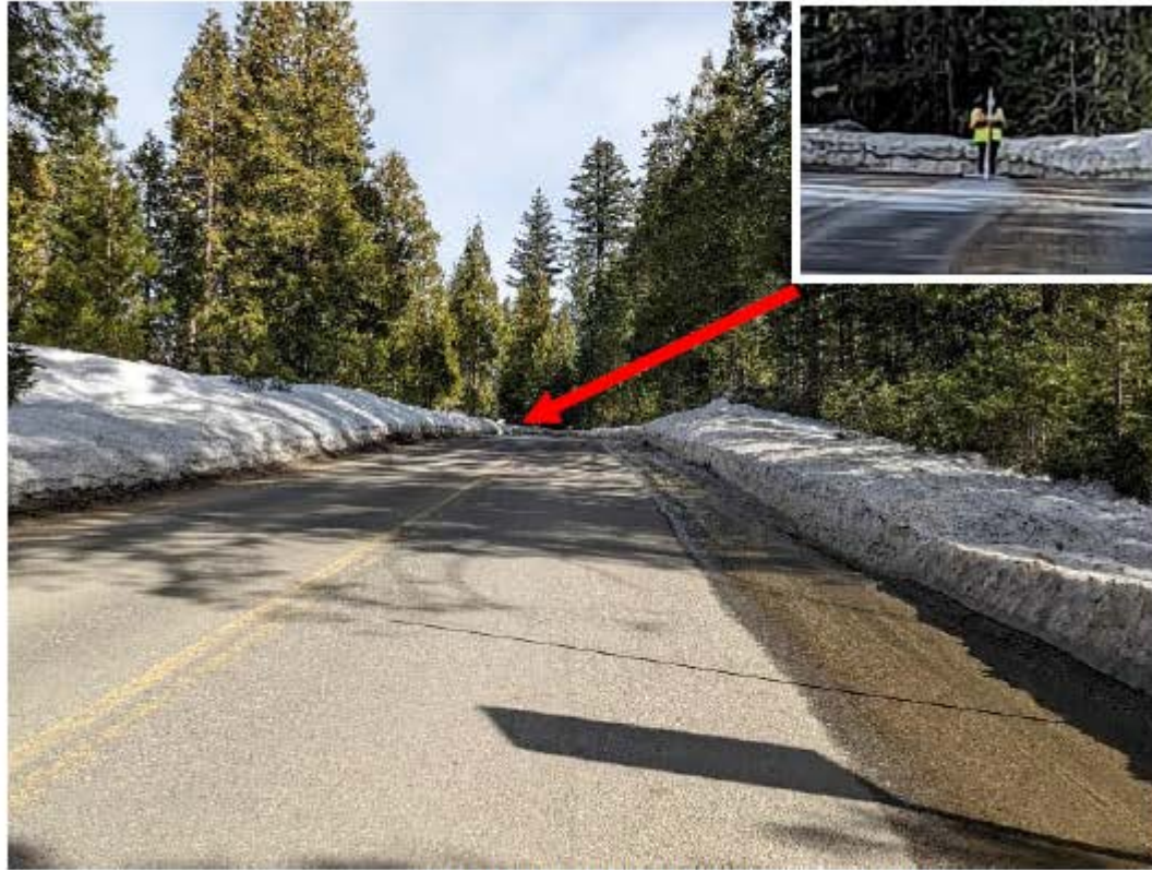
Traveling East Towards Project Driveway
