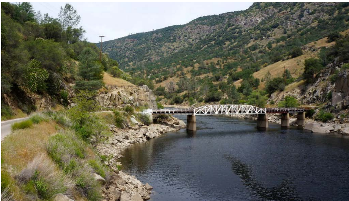
Photo 1. Italian Bar Bridge over Redinger Lake
