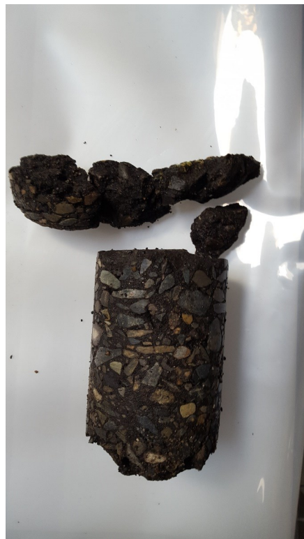
Core C-8 NB Left Lane, Sta: 386+80
