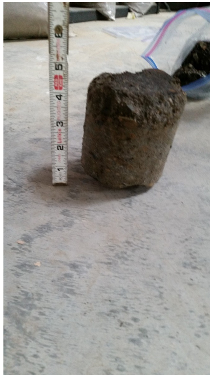
Core C-10 NB Left Lane, Sta: 554+80
