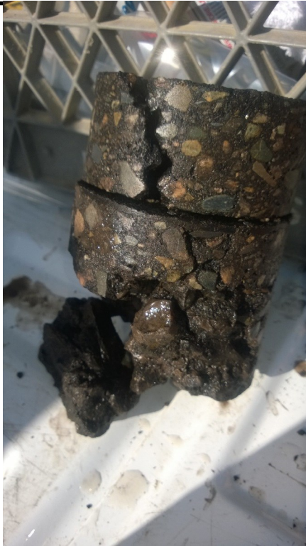
Core C-3 SB Right Lane, Sta: 295+10
