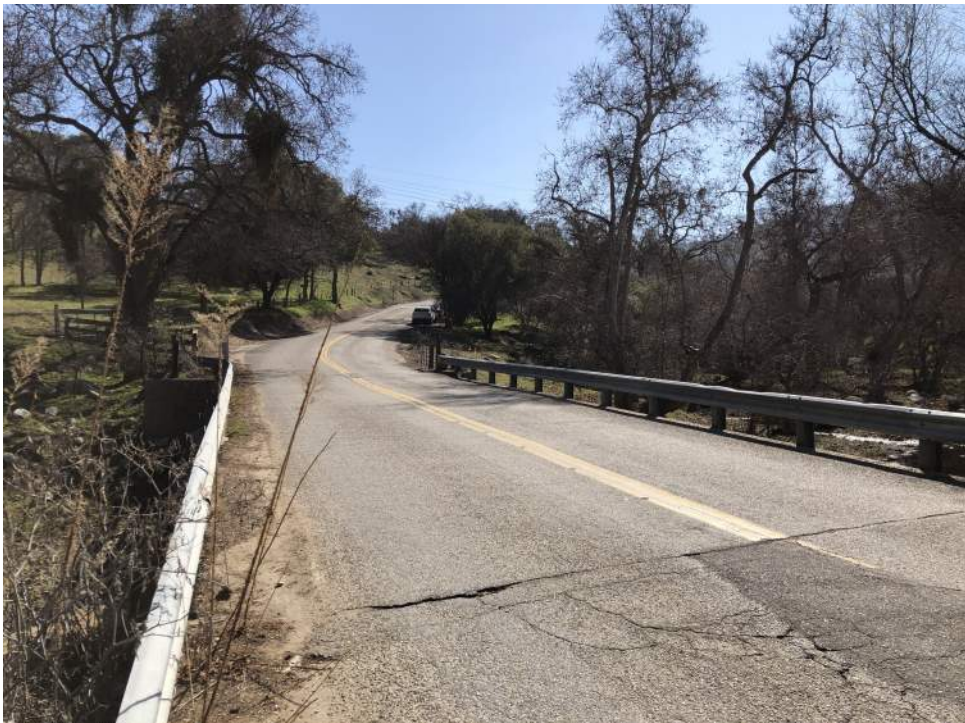
Figure 2 View of the project looking towards Burrough Valley Rd, facing southeast.
