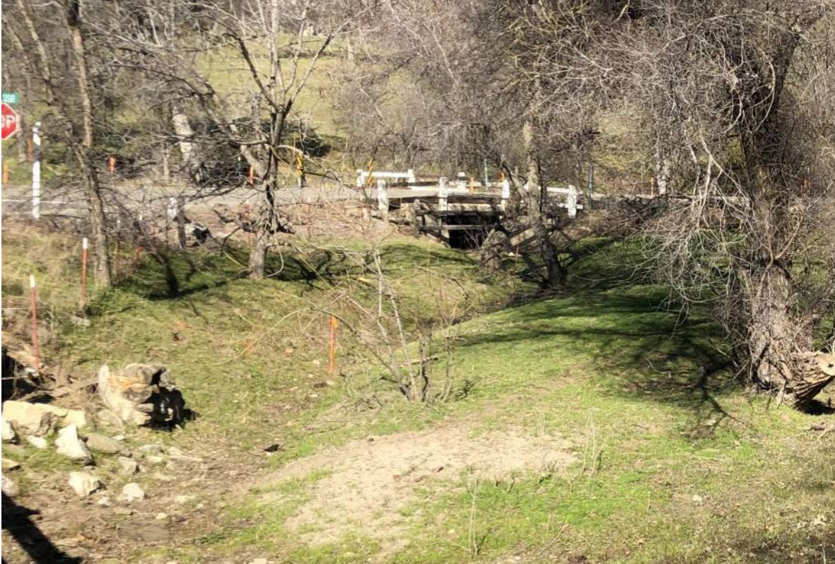
Figure 5 View of the existing culvert on Tollhouse Rd.
