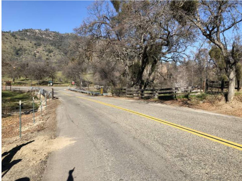
Figure 1 View of the project on Burrough Valley Rd, looking towards Tollhouse Rd facing northwest.
