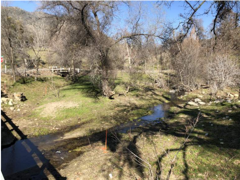
Figure 3 View standing on the bridge, looking upstream.
