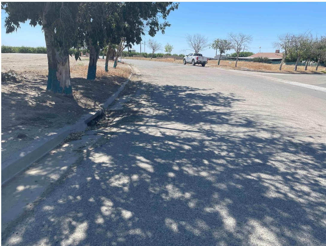
Photograph near core location C-1 along Progresso Avenue – Sinking drainage inlet
