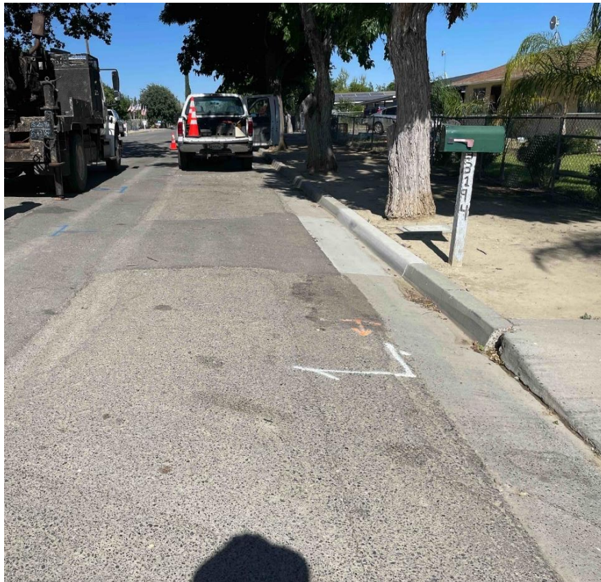
Photograph near Core Location C-4 along Hidalgo Avenue - Note differential movement cracking of concrete curb
