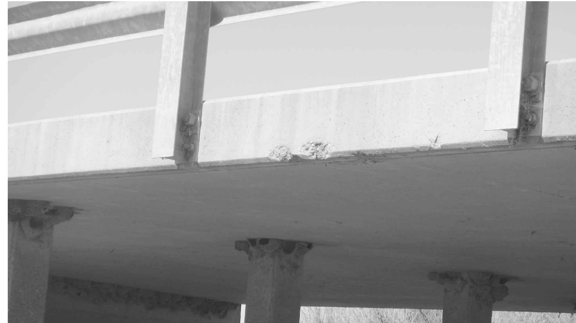
SPALLS ALONG SOUTH EDGE OF DECK
