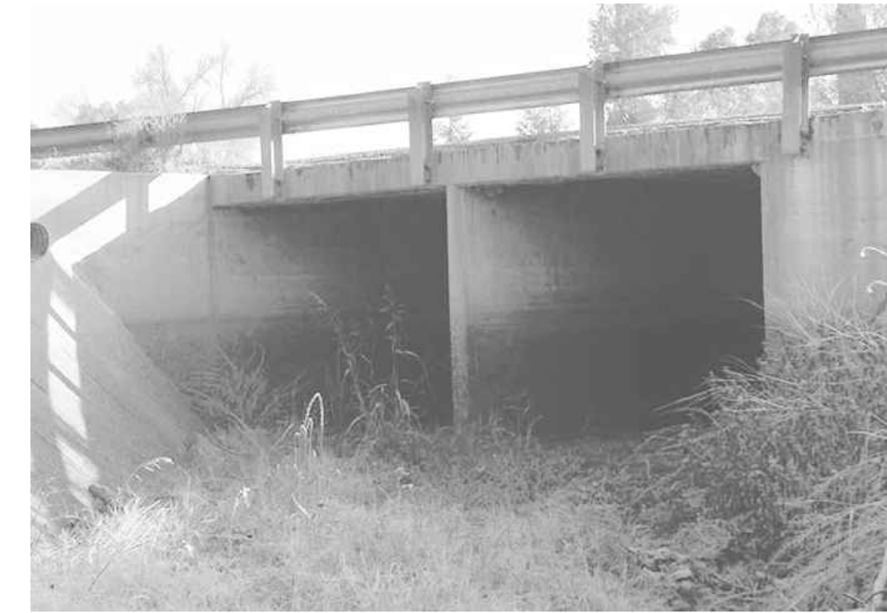
ABRADED CULVERT WALLS
