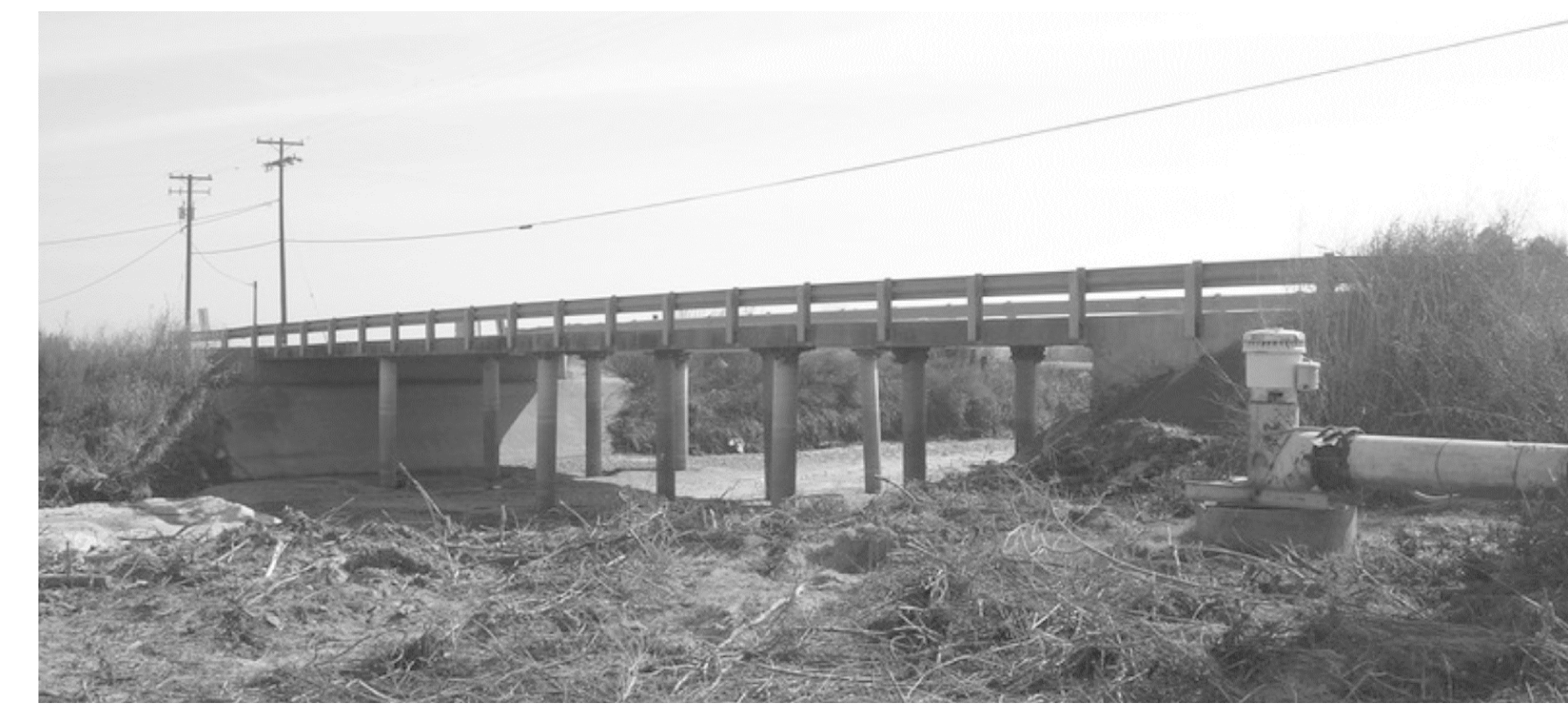
ELEVATION LOOKING SOUTHEAST
