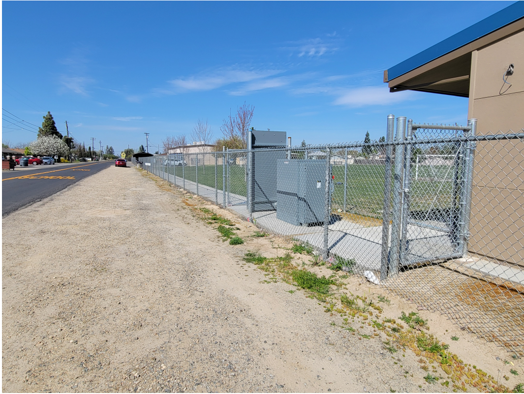
Figure 7: North side of Clemenceau Ave facing west near the elementary school.
