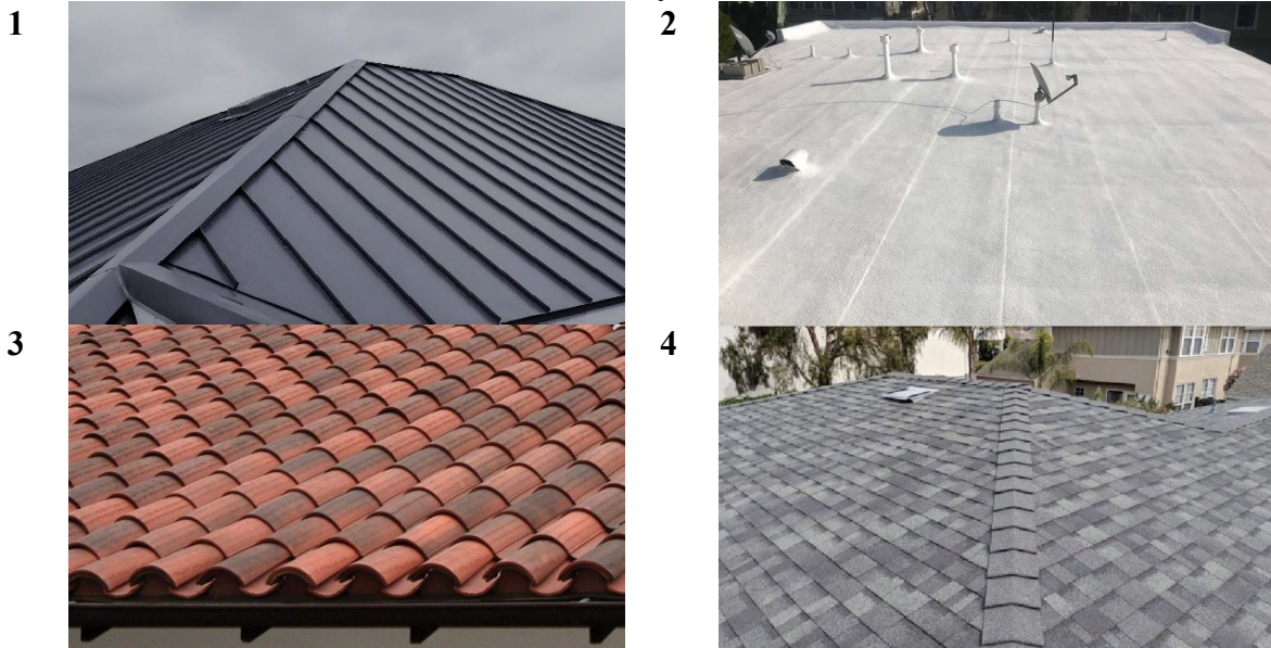
Figure 4-5 Allowable Roof Materials
